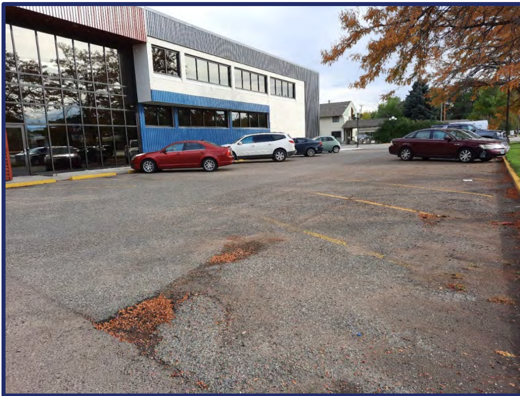
Figure 8. Tribal Administrative Office
